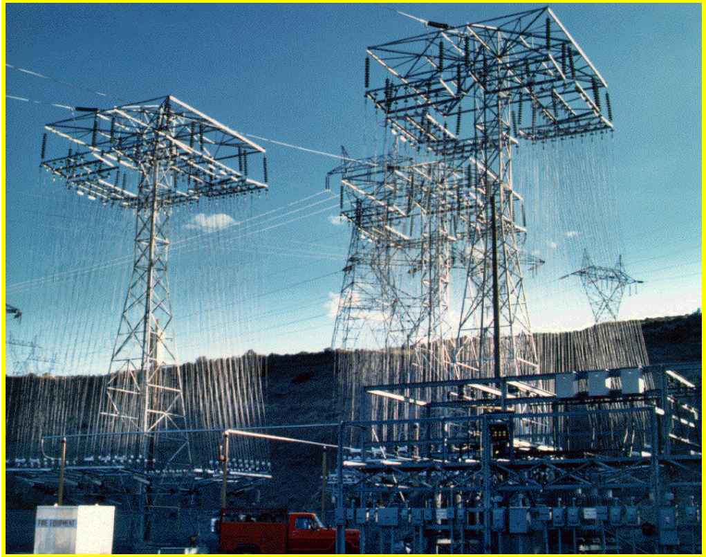
Figure 7-19 The BPA Braking Resistor
